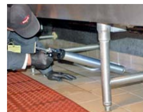
Apply DeTour beads with the optional refillable applicator gun
