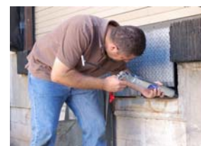
Apply DeTour beads from 10 oz. cartridge and caulking gun
